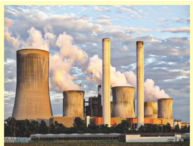
The 1,100 MW Karachi Nuclear Power Plant unit 3 (K-3)
