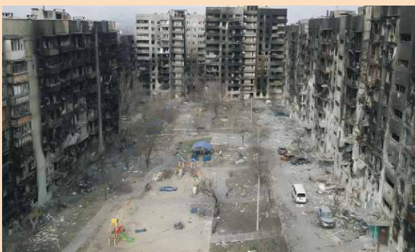
An aerial view shows residential buildings that were damaged during the Ukraine-Russia conflict in the southern port city of Mariupol, Ukraine
